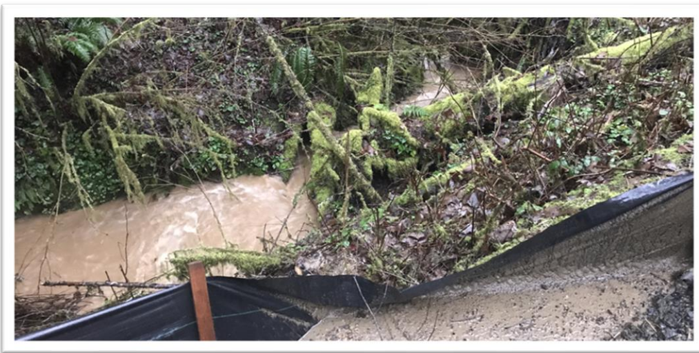
Photo 2. Example of other measure, sediment trapping using silt fencing.
