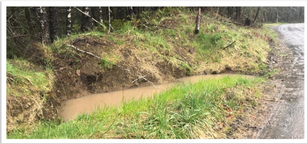
Photo 1. Example of other measure, settling basin.
